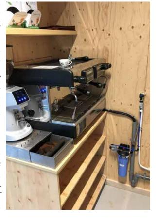
After a search, they finally arrived at Watts and its innovative scale control system OneFlow®. The compact OneFlow® version with a flow rate of 4 liters/min, suitable for protecting a separate unit, ultimately proved to be the ideal solution. Indeed, OneFlow® does not add salt or chemicals, but thanks to its innovative operation based on TAC media, the water composition, especially hardness and Ph value, remains unchanged.
